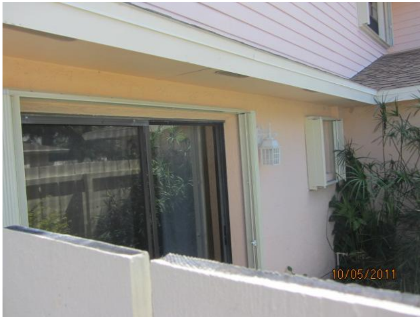
Accordions covering all sliding glass doors
